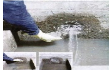
Water plug used as a dry powder mix, the water incoming will provide the moisture to cure the water plug. Water plug can also be pre-mixed but speed is essential.
