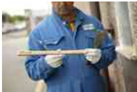
5. Timber pieces can be supplemented in deep recessed areas
