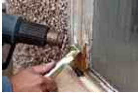
1. The worst affected rotten wood and debris is removed
