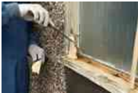
4. Apply the epoxy to work area and shape as required.
