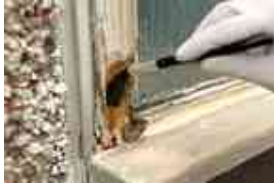
2. EWS is brushed on to stabilise the remaining timber.
