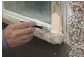
6. The complete area is finished ready for painting
