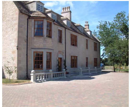
Stretton Hall on the border of Lincolnshire and Leicestershire, refurbished to a high standard using many of Construction Chemicals products. The cellars have been waterproofed using tanking slurry and have been converted into a gym, sauna and plunge pool.
