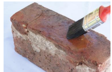
Apply two coats of Super Seal by brush or spray for long lasting protection.
